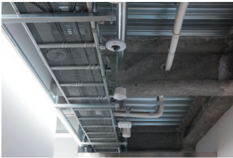
Figure 23: Ceiling with exposed piping
