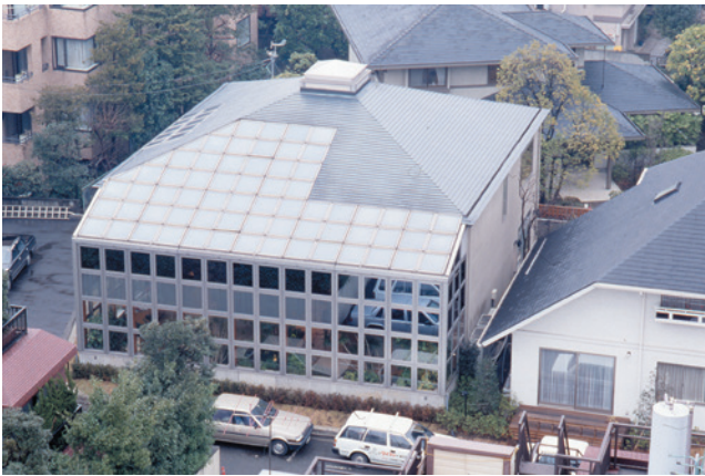
Figure 1: Full view of the south side of the TRON Intelligent House. The indoor and outdoor environmental/weather sensors constantly measure temperature, humidity, air pressure, wind speed, wind direction, rain fall, illuminance, etc. All the windows, including those in semi-outdoor space, are automatically opened and closed by computer control based on these measurements.
