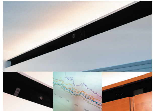
Figure 55: To install 150 sensors without performance degradation and without presence, black slits were created around the folded ceiling for installation
