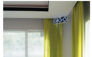
Figure 40: Adjusting temperature unevenness with a circulator
